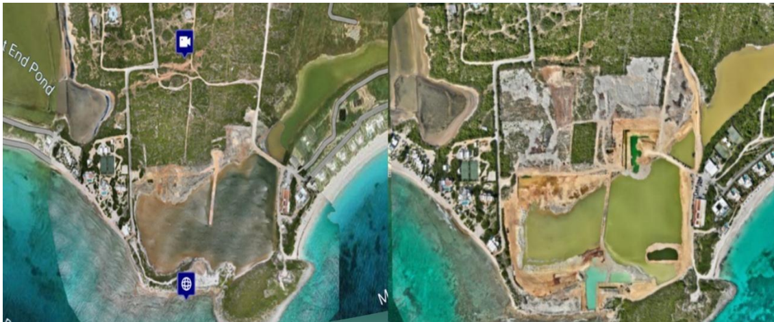
Figure 20. Orthomosaic comparison of Gull Pond (2024 – left; 2026 – right) showing significant land development, excavation, and expansion of artificial water bodies associated with the Port Nimara Marina project.
